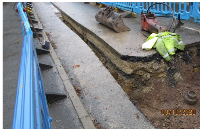
Milton Street roadworks, October 2020
